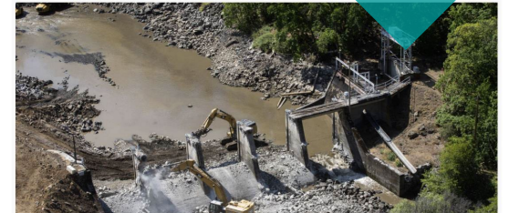
Copco 2 Deconstruction Begins on Klamath River
